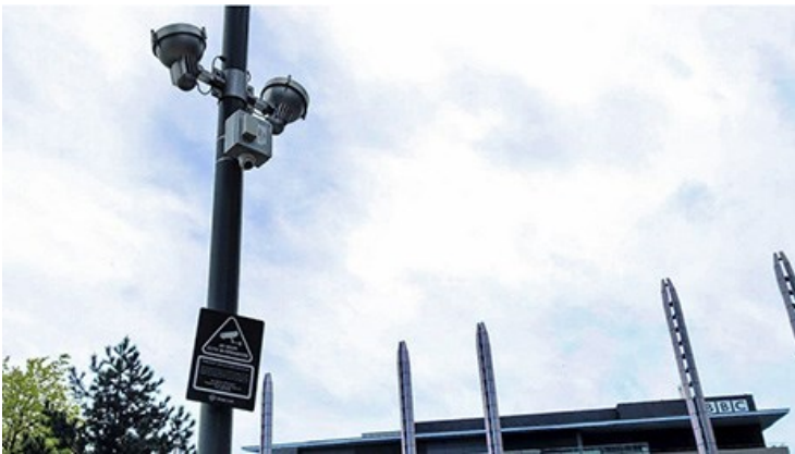
Particle counter in use for air quality monitoring in the UK
